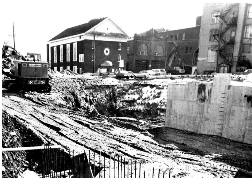
Fig. 6. Demolition of the Bank Street Synagogue and the Old Fire Station. Photo courtesy of Rabbi Jeremy Schwartz, Temple Bnai Israel, Willimantic, CT.
