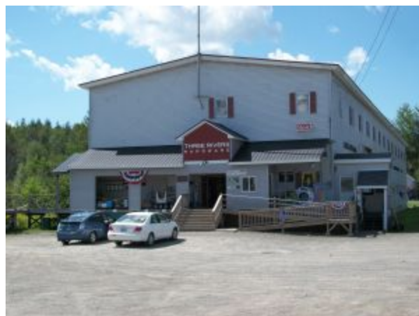
The former ATCO Spool Mill in Milo, Maine, now a hardware store. Photo by Jamie Eves.
