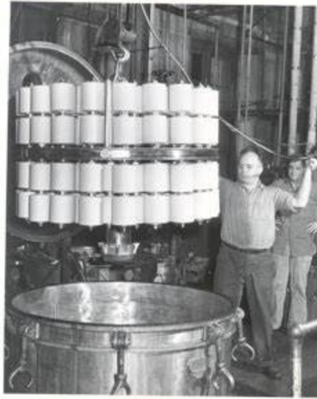
Pressure dye vats like this replaced inefficient open dye vats in the 20th century. Using a pressure dye vat, a worker could dye thread right on the spool. This photo was taken c. 1950 at the American Thread Company's Willimantic mills. From the collections of the Windham Textile and History Museum.
